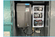
Smart inverter Strong low-speed torque with stable operation down to 0.01 Hz, ideal for heavy-load start and frequent speed changes.
